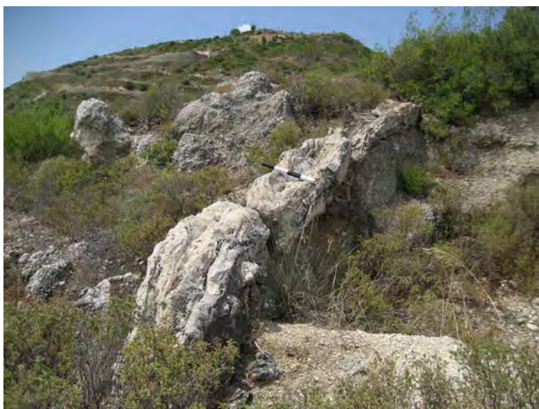
Fig. 2. Carbonate sinter deposits from the aqueduct of Sikyon at Sesi. The deposits are at least 40 cm thick, and nearly completely filled the ancient channel. At this site, the walls and cover of the aqueduct have disappeared, and only the channel fill survives (Y. Lolos).
